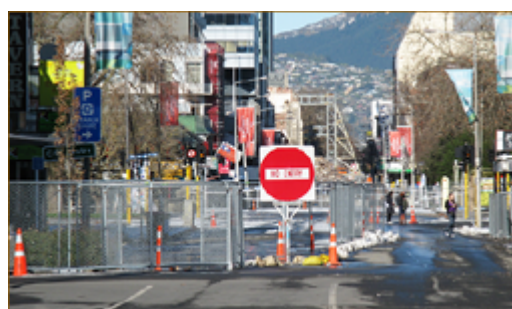
Figures 1 & 2: Bus crushed by masonry facade & part of the Christchurch central business district cordoned as of August 2011.
