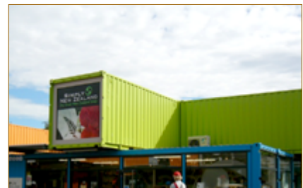
Figure 3: Offices in the temporary Westpac business hub & stores in refurbished shipping containers in the Christchurch CBD, Re:Start Mall.
